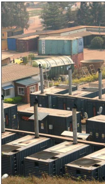
Diesel powered generators in Gikondo Valley in Kigali supplement the shortfall in the electricity supply from mainly hydropower sources that are still not able to meet the rising demand levels.
